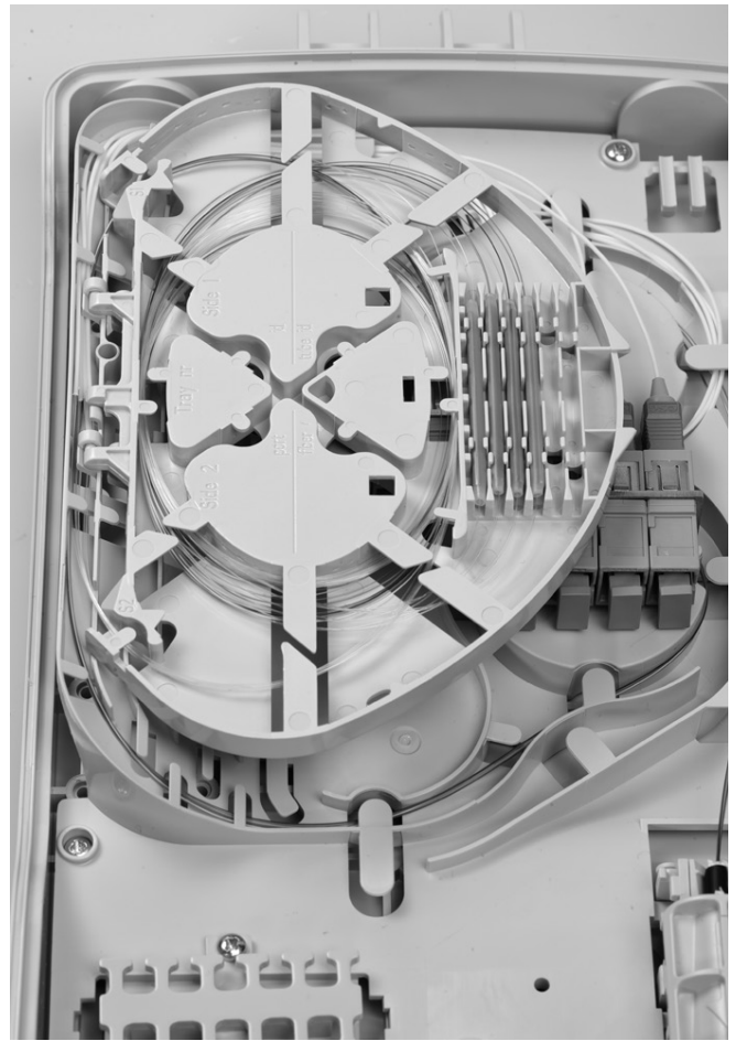
4.8 Splice the fibers from the feeder cable to the pigtails and store the overlength into the tray.
