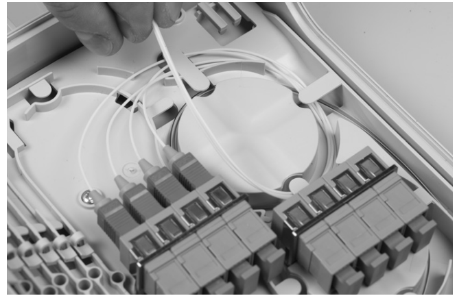
4.4 Connect first four 900µm pigtails.
