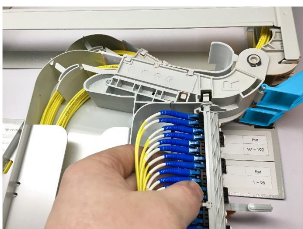
10.4.7 Patch the connectors into the adaptors.
